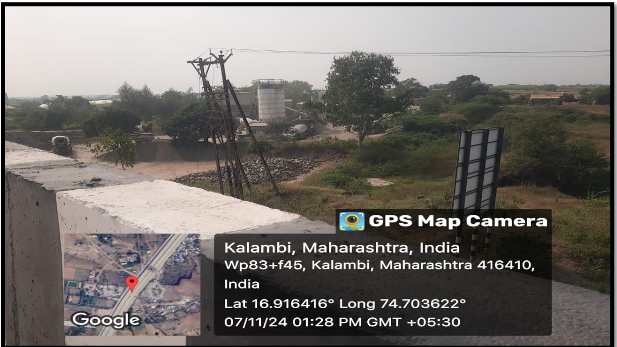
Pictures dated 07.11.2024 showing that RMC unit of Respondent No. 2 is operating illegally.
